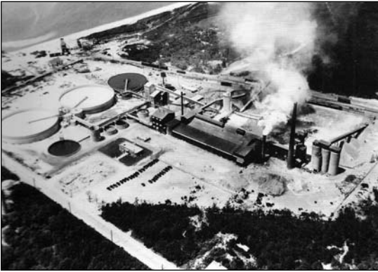
Cape May Magnesite Plant, 1942.
